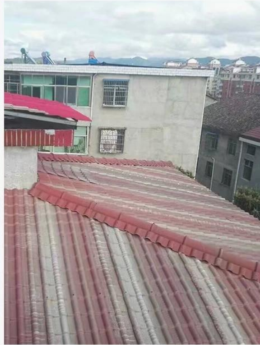
Inferior resin tiles are easy to fade
