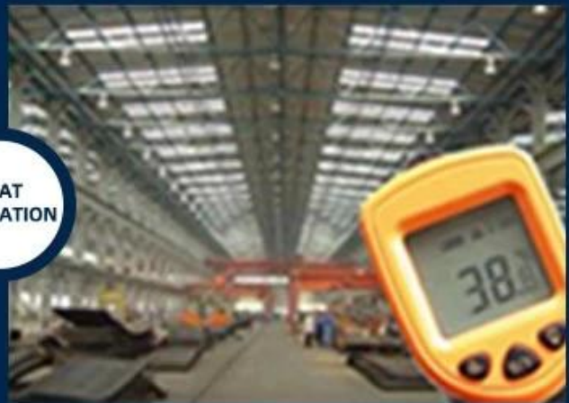
Direct sunlight iron tile Temperature too high
