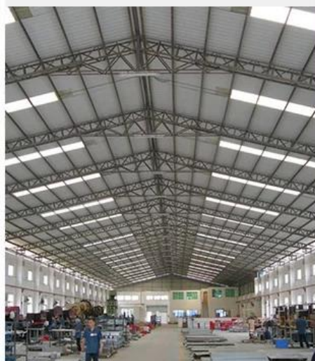
Large factory area
