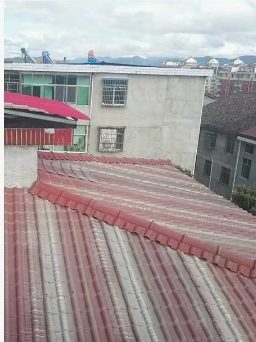
Inferior resin tiles are easy to fade
