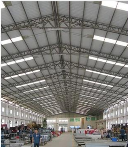
Large factory area
