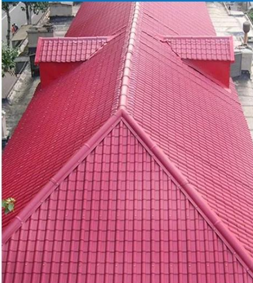
Renovation of old houses in Guangzhou
