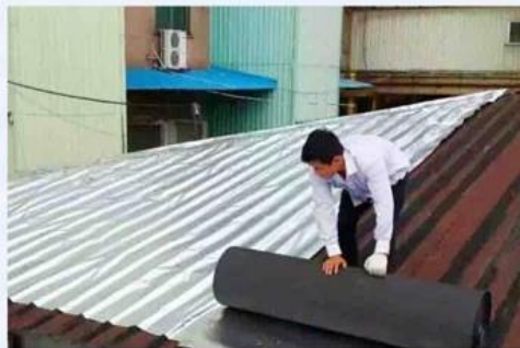
Iron tiles are not soundproof
