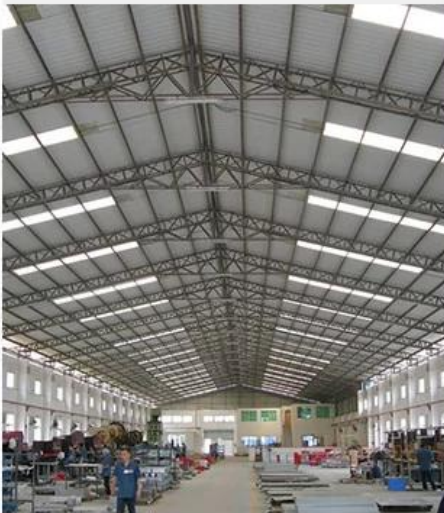
Large factory area
